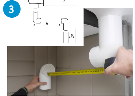
3 Determine the offset length (A) using Fig 2 allowing for depth of socket and taking into consideration the downpipe bracket distance from the wall (B). Cut downpipe as per measurements.
