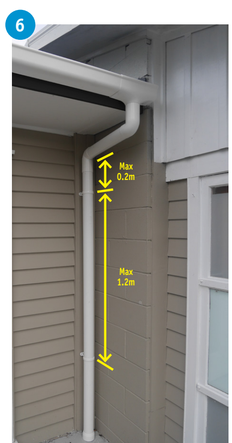
6 Connect downpipe to access pit, surface drainage or stormwater outlet (as shown in photo).
