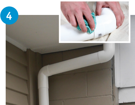
4 Solvent cement all remaining elbows to downpipe on ground, before completing offset installation.
